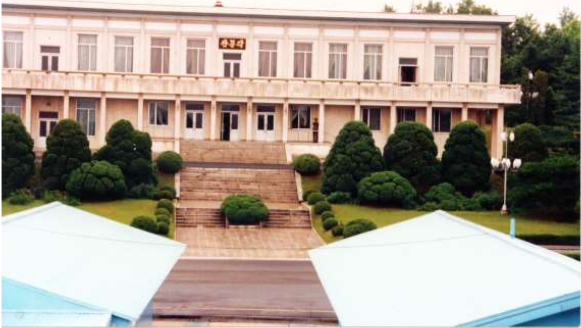
Building facade on the North Korean Side. A North Korean Army officer is observing with binoculars
